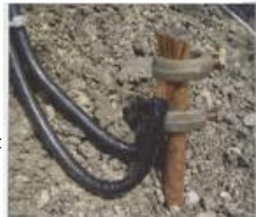
A: 12 Ga is fine (bigger is always better but 12 Ga will get the energy started in the correct direction; the NEC Code wants 8 Ga) and will do a decent job of keeping lightning fingers from flying around and moving into the house looking for gas/water pipes when the copper ground rod outside gets saturated/overwhelmed in trying to dissipate a big stroke's current (could be thousands of Amps)
